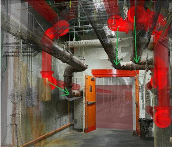
Figure 3.5. 3D laser scanning an information model used to coordinate 27
